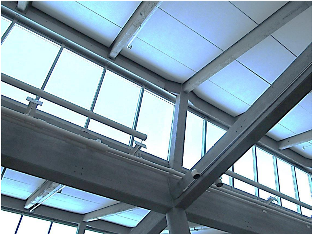
1. Atrium view of Roof Beam at top of Clerestory Window
