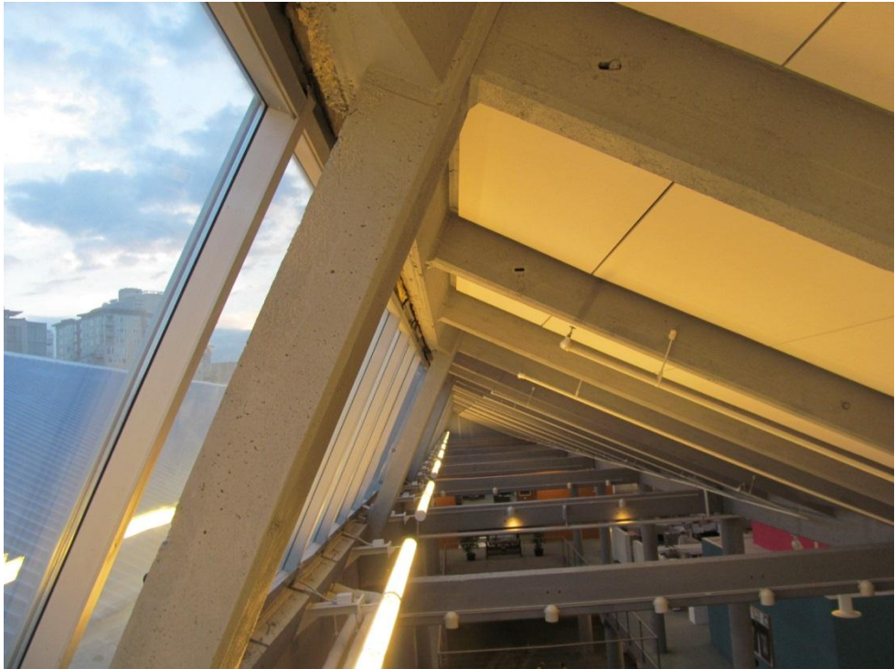
2. View Along Length of Beam
