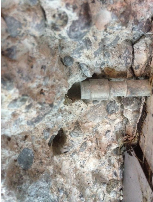
5. Exposed Window Connection Anchor Bolt
